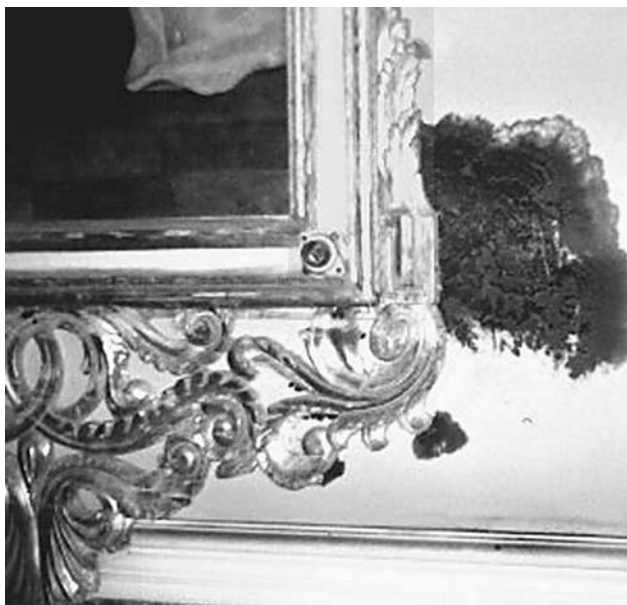
Figure 4.3. Fungal growth behind a painting hung on a church wall in Salvador, Brazil. Photo: Dr Fatima Bento.
