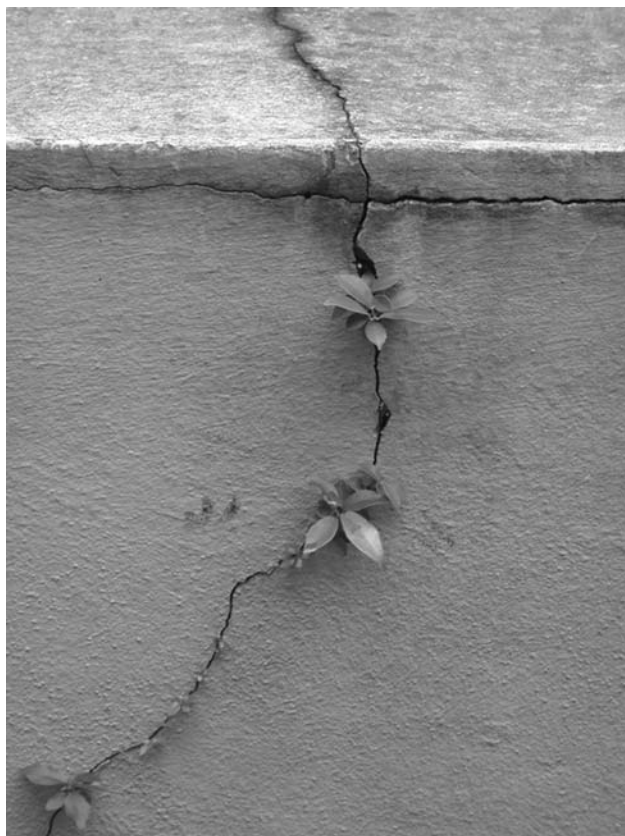
Figure 4.12. Seedlings of higher plants growing in a crack in a wall in Porto Alegre, Brazil. Root pressure will soon enlarge the crack. Photo: Dr D. Allsopp.
