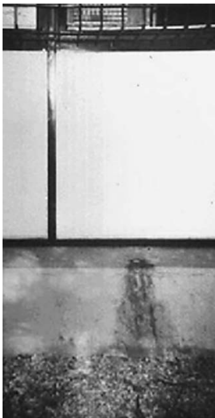
Figure 4.7. Leakage of air-conditioner condensate encouraging biofilm formation. Photo: Dr Christine Gaylarde.
