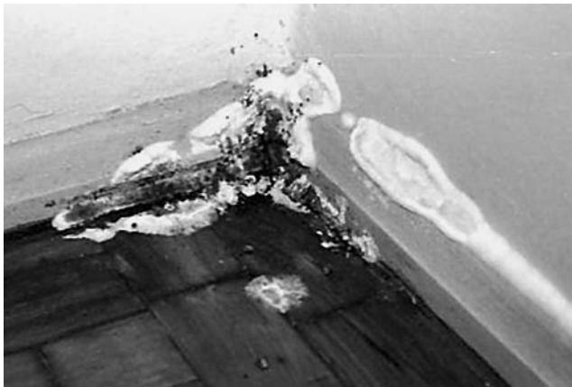
Figure 4.1. Dry rot: developing fruiting bodies of Serpula lacrymans on wall, painted-wood skirting board, and wood-block floor. Photo: Dr Christine Gaylarde.
