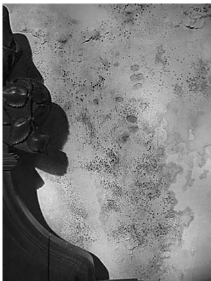
Figure 4.2. Mould growth on a painted church wall in Wiltshire, UK, caused by a leaking drainpipe which is wetting the wall from outside. Photo: Dr D. Allsopp.
